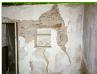
Interior restoration of the small room in the east corner of the Knapp farmhouse revealed this small window which had been covered with plaster. The discovery indicates that at one time this was an exterior wall.
