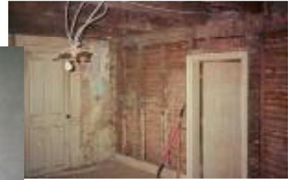
Above: The "naked" parlor striped of flaking plaster and water damaged ceiling.
