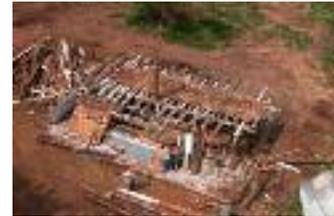
In April 2008, MTHS contracted with Hartland Restoration, Inc. to dismantle the barn and salvage the framework and floorboards. This timber will become the basis for a planned Visitors' Center on the property. The original concrete floor and cow stalls will be retained and used for demonstrations of life on the dairy farm. The framework is currently being stored on the floor of the old barn.
