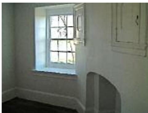
One of four second floor bedrooms sports a gleaming new coat of plaster and restored windows, ceiling and floor.
